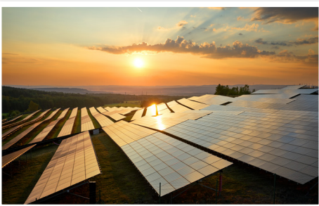
Compatible with BYO Solar Installs
