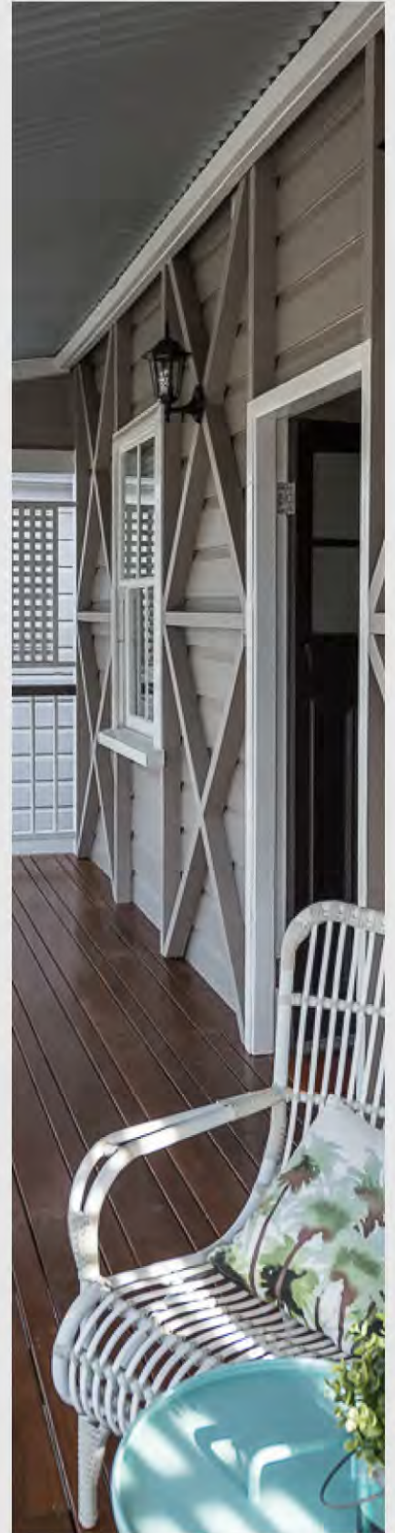
Verandah exposed timber frame. 1
