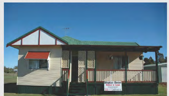
Mitchelton finished on site . 1
