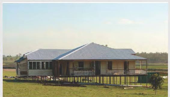
Millwood new roof and restumped at Boonah. 1
