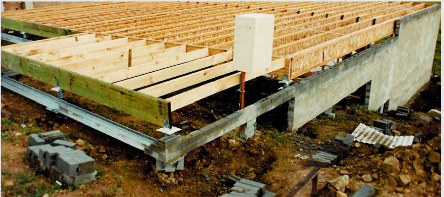
Suspended Timber Floor. 1
