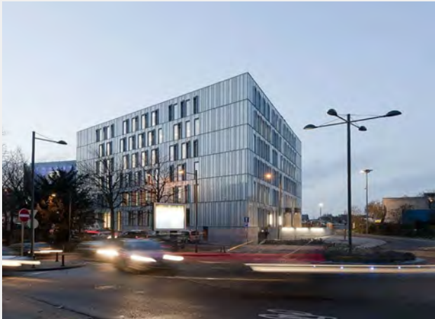
Architectes Associés, Aeropolis II, medium, 1485x 976, Belgium, Schaerbeek, 12/06/2020 accessed , https://www.circularfacades.com/aeropolis-ii .
