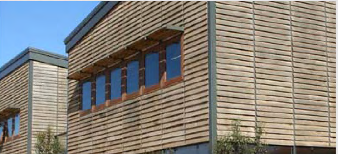
Natural Edge Weatherboards 1
