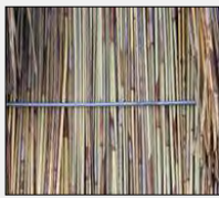
Figure 25. Galvanised wire sway of min 3.15mm
