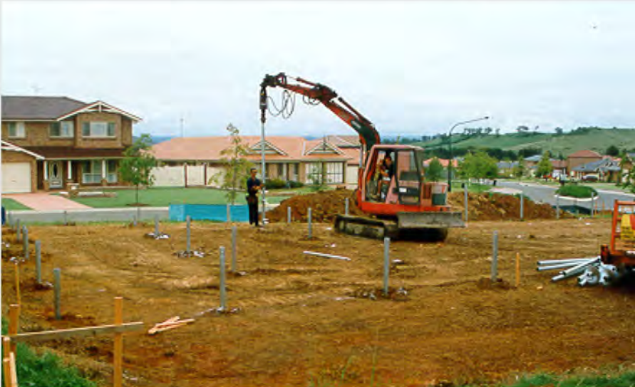
Screw-in steel piles 1
