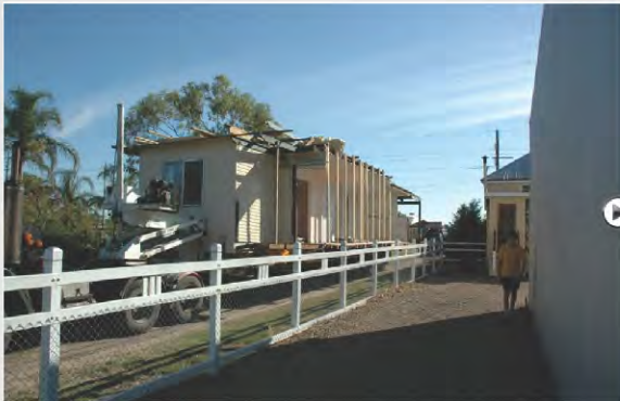
Mitchelton relocating to new site in Dalby. 1
