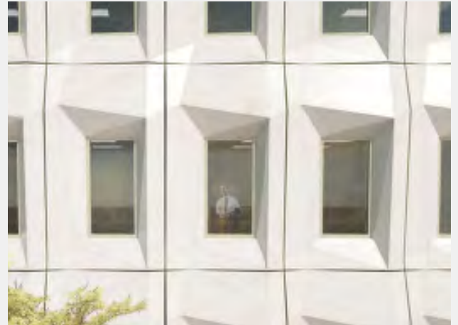
"BioBuild: structural façade panel in biocomposite materials." CIRCULARITY IN THE BUILT ENVIRONMENT: CASE STUDIES (United Kingdom: Ellen MacArthur Foundation, 2016), 48.
