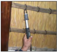
Figure 24. Correct binding tension.
