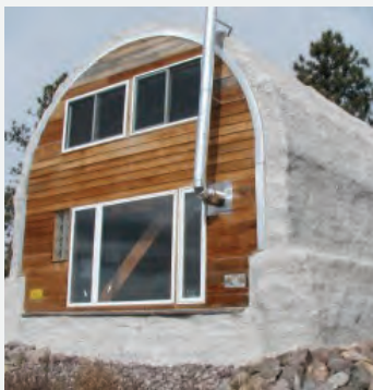
Figure 10: Papercrete - The Carriage House by Kelly Hart located in New Jersey. Source: Hart, Kelly, "Papercrete," (Kelly Hartworks LLC, established in 2001), http://www.greenhomebuilding.com/papercrete.htm
