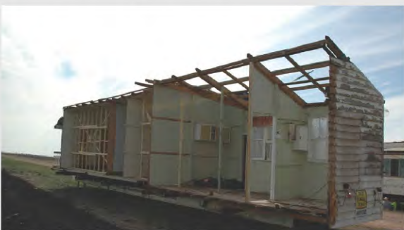
Millwood loaded undergoing removal works. 1
