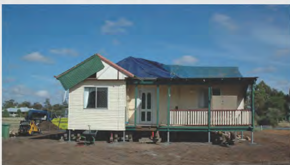
Mitchelton being stumped on site in Dalby. 1
