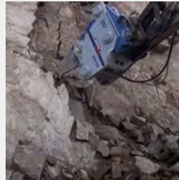
2.Drill Excavation of sandstone by drill
