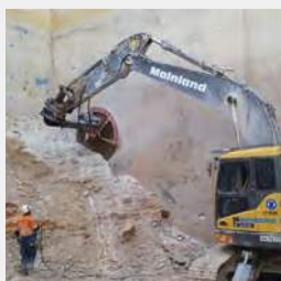
1. Crushing Crushing loose material for road base
