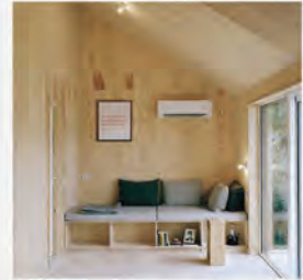
4. Finishing Plywood is finished with satin polyurethane for walls and hard finish oil polyurethane for flooring. Install prehung interior doors and trim moldings.
