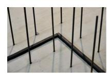
Both, straight and angle joints need to be butt jointed. The joint areas must be form-fit in order to avoid any discontinuity in the system.
