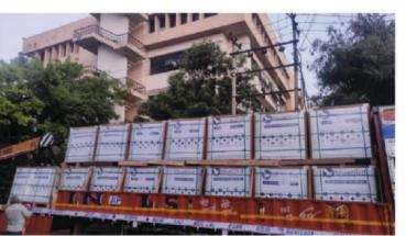
Panels are received with not more than 2 Pallets stacked Vertically.
