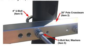
9. Orient the crossbeam where the top of bracket will be located on the pole as shown below
