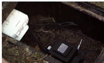
POSITION YOUR LOW VOLTAGE TRANSFORMER
