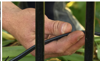
RUN LOW VOLTAGE CABLE
