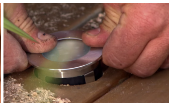
COMPLETE INSTALLATION OF LIGHTS
