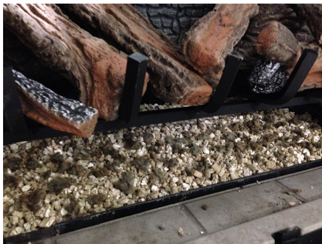
Figure 21 - Completed Installation of Vermiculite and Embers
