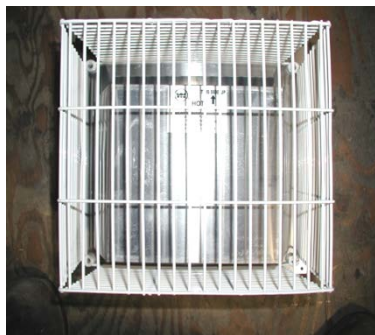
VIEW OF SAFETY CAGE
