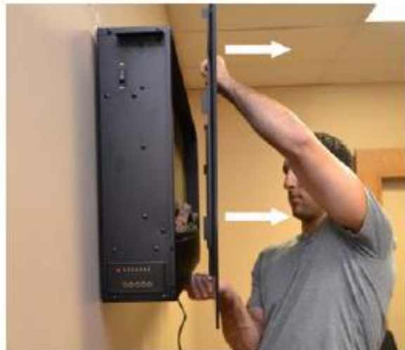
b. pull glass panel away from wall
