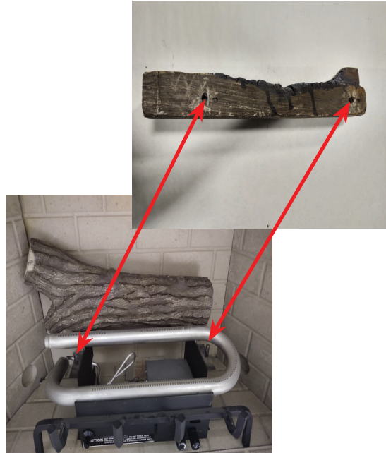
Figure C - Middle Log Placement
