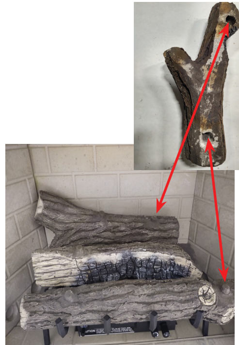
Figure G - Top Right Log Placement
