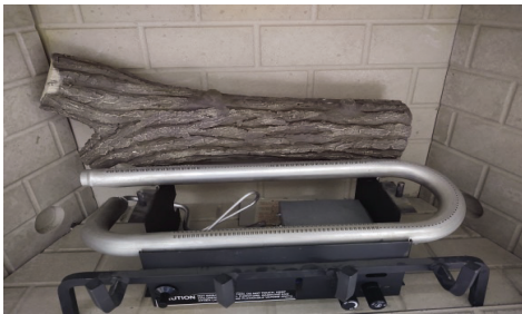
Figure B - Install Rear Log
