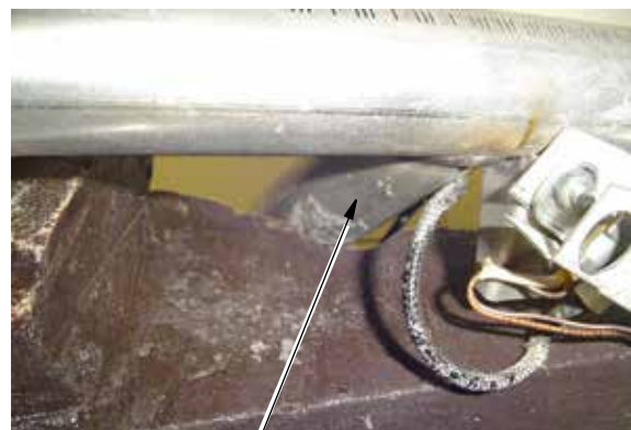
Figure 17B - Installing Back Left Log (D-018) Rear View
