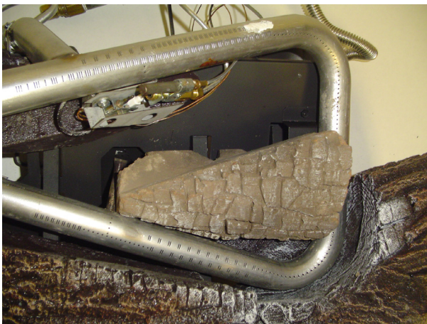
Figure 21A - Installing Charred Log Top View
