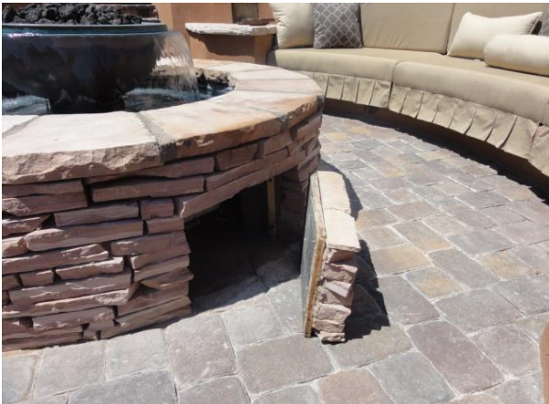
Stone enclosure on site
