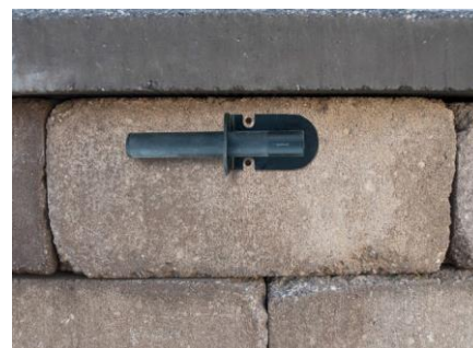
Figure 6.4 – Dry fit the bracket
