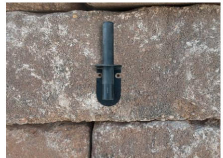
Figure 6.8 – Dry fit the bracket
