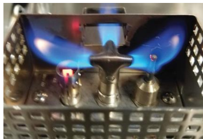
Figure 9.2 – Pilot flame coverage of thermocouple.
