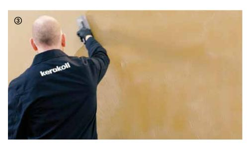
→ Apply the 2<sup>nd</sup> coat once the material has hardened (3 - 12 hrs).
