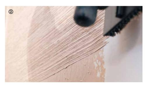
→ Pass over the wet strip with the Stripe tool while the product is still fresh, creating horizontal lines, making sure to keep the geometry parallel with the plane.
