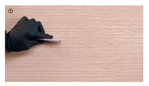
→ Lightly sand by hand in order to remove any small flaws or lumps before applying **Decor Paint**.
