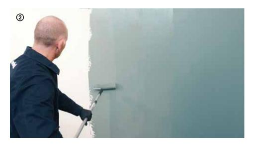
→ Decor Paint must be carefully applied with a roller over the whole surface in 2 coats, either pure or diluted to a maximum of 5 - 10%.
