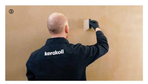
$\rightarrow$  Remove any dust with a dry flat brush or a cotton cloth and then apply the 2<sup>nd</sup> coat of **Finish**.
