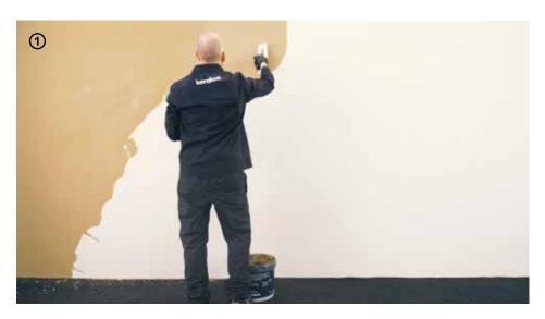
→ Apply the 1<sup>st</sup> coat of **Patina**® smoothing the product with small and even strokes of the spreader over the entire surface.
