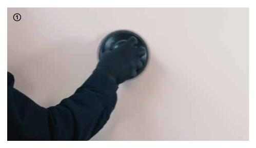
→ Before applying **Decor Paint**, sand the surface with 80 - 220-grain sandpaper in order to make the surface perfectly smooth and pleasing to the touch.
