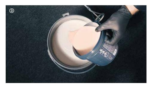
Tip: in order to improve the visibility of the processing, Wallcrete in paste form can be coloured by adding a few drops of Decor Paint of the same shade as the final colour.
