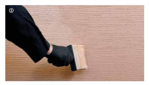
→ **Decor Paint** must be applied over the whole surface, by brush, in one or two coats, either pure or diluted to a maximum of 5 - 10%, following the direction of the horizontal lines.
