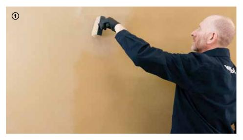
→ Once the coloured texturizing finishing coat **Patina**® has completely dried, apply the 1st coat of **Finish** by brush without sanding.
