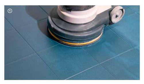
→ The **Microresina® Zero** supporting layer must be carefully prepared: sand with a sander or floor buffer with **Carboplus Sic 220** abrasive pad to even the surface; clean thoroughly with a vacuum in order to remove all sanding residues.
