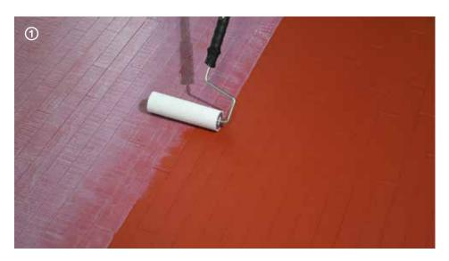
$\rightarrow$  Evenly apply **Microresina® Xtreme** with **Roller Plus** respecting the coverage of  $\approx 80 \text{ ml/m}^2$ .
