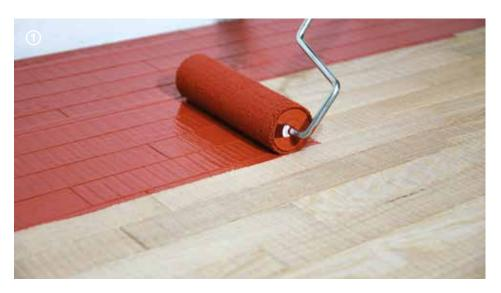
$\rightarrow$  Evenly apply the 1st coat of **Microresina**® with **Roller Plus** respecting the coverage of  $\approx$  110 g/m².
