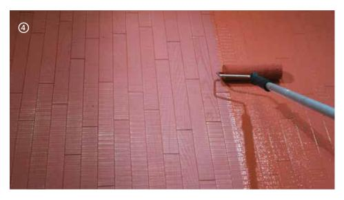
$\rightarrow$  Evenly apply the 2<sup>nd</sup> coat of **Microresina**® with **Roller Plus** respecting the coverage of  $\approx$  110 g/m².
