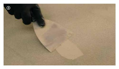
$\rightarrow$  Before the application check that **Floorzero**® has no defects and imperfections and that the **Net 90** mesh is not showing.
