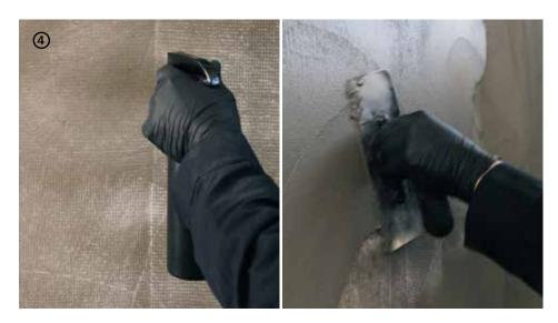
→ After ≈ 3 hours, dampen the 1st coat of **Wallzero®**, then apply a second coat smoothing the product with small strokes of the trowel in order to obtain a flat and even surface.
