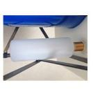
Step 8 Put liquid hand soap in the soap dispenser and screw it to the bottom of the counter. Put the soap dispenser pump through the hole on the right side of the counter top.
