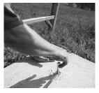
**5.** Use the 15/16" socket wrench to tighten the nut on top of the anchor.
