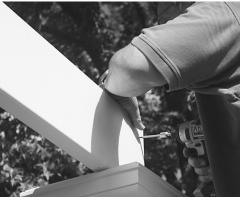
the outside of the aluminum angles on top of the columns using the 2.5" hex head stainless steel screws. Set the clutch on the drill so the screw is not stripped.
