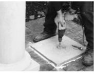
**2.** Use the hammer drill and 5/8" masonry bit to drill a 5" deep hole.
