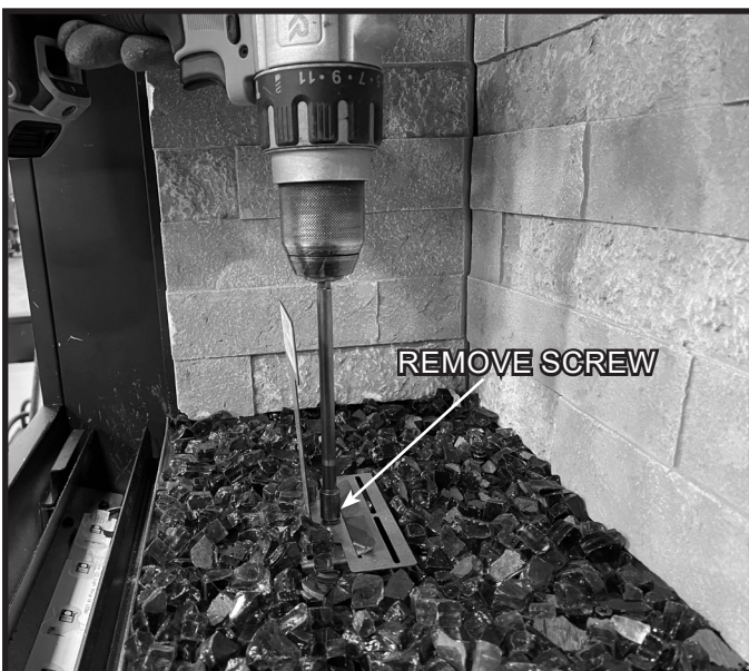
Figure 11.4 Place Media, Remove Media Placement Jig Screw
