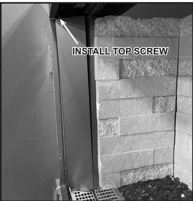
Figure 11.21 Transition Panel installed
