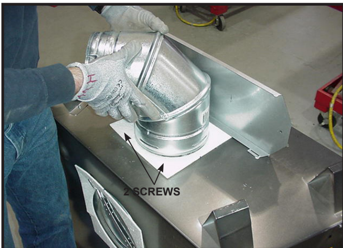
Figure 6.8 To attach the first section of vent pipe, make sure to use the fiberglass gasket to seal between the first vent component and the outer fireplace wrap. Use 2 self tapping screws to secure the gasket to the outer wrap.
