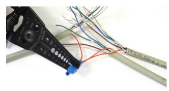
6. Double check that the 3 drain wire/bare wires are also crimped together as this is what continues the shielding throughout the network. The shielding and drain wire MUST be connected to Earth Ground at **only one point** of the cable run.
