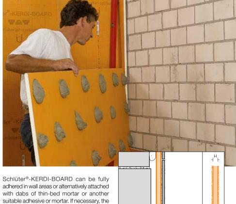
Schlüter®-KERDI-BOARD can be fully adhered in wall areas or alternatively attached with dabs of thin-bed mortar or another suitable adhesive or mortar. If necessary, the material may be secured with additional wall anchors. In the case of stud frames made of wood or metal, Schlüter®-KERDI-BOARD is attached with screws from the matching hardware system.
