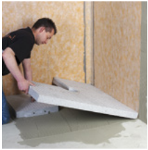
Re 1. and 2. Set levelling board in place, if required.
