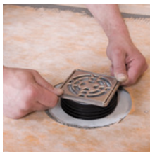
Re 9. Insert the stainless steel grate and frame at the appropriate height as part of the installation
