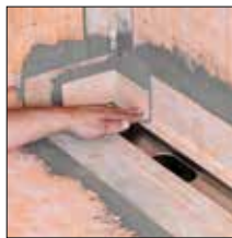
For 3. Adhere KERECK interior corner
