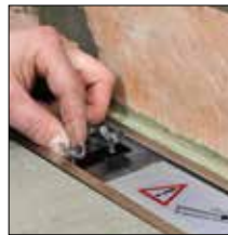
For 2. Use height adjustment aid to match frame...
