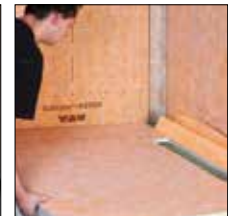
Fig. 3. Slide the sloped tray under the edge of the channel body
