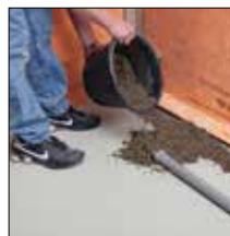
Fig. 6. Apply sloped screed
