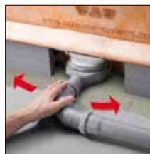
Fig. 5. Align the drain pipe
