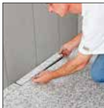
For 6. Adhere covering – leave the area of the covering support open when applying grout
