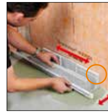
Fig. 1. Align the channel support
