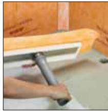
Fig 2. Insert drain pipe
