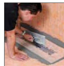
Fig. 4. Adhere Schlüter®-KERDI collar with Schlüter®-KERDI-COLL-L
