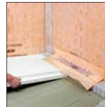
Fig. 3. Evenly install the levelling board
