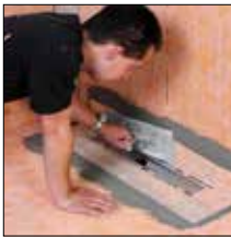
Fig 4. Adhere KERDI collar with KERDI-COLL-L
