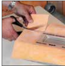
For 1. Cut the KERDI collar to size
