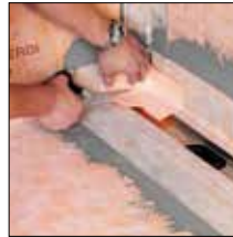
For 2. Adhere KERDI collar/ cut KERECK interior corner to size
