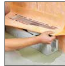
Fig. 2. Insert the channel body
