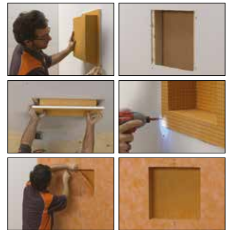
Installation in drywall
