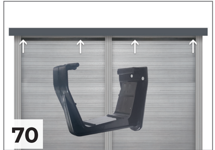
70 Attach gutter clips placing them evenly. Make sure they are level. You may also create a slight slope in the direction of running water.
