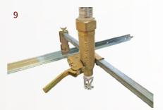
Slide the outlet reducer into the center bracket.
