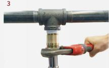
Connect the nut of flexible hose to the inlet nipple using a pipe wrench. DO NOT use PTFE or pipe joint compound on the inlet nipple at the hose side since there is already a seal gasket in place to seal the joint. Tighten the connection to a maximum torque of 15 ft-lbs/20 N\*m. Too much torque may cause damage to the seal gasket.
