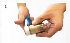
(A) Pipe side: Apply PTFE thread seal tape or pipe joint compound to the tapered threads of the inlet nipple.
