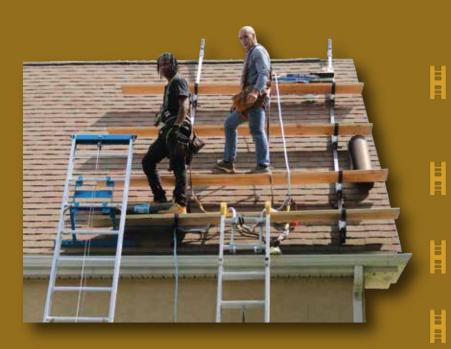
Each rail is 21ft standard (2x 8ft sections, 1x 5ft section) & extendable to 42 ft.
