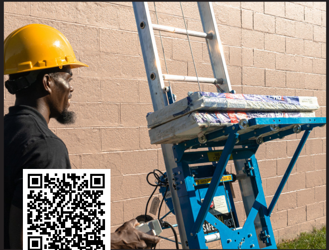
Electric Material Hoists
