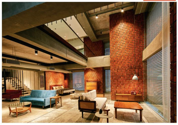
the designer has used exposed brickwork in the façade which adds to the visual element of the store. The exposed brick masonry and block masonry are laid vertically instead of the conventional horizontal pattern. This play of different texture of planes defines the areas instead of having walls to divide the space.
