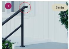
Remove the top rail end cap, and insert the adjustable connector.
