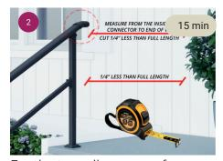
For the top rail, measure from inside connector to wall. For middle rail, measure from post to wall. Cut the measured length minus 1/4" for both rail.
