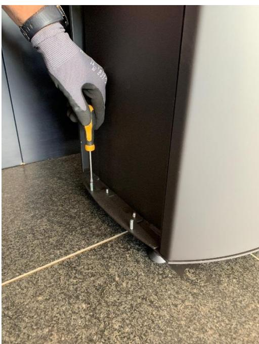
3. Now screw two of the threaded pins (M5 x 20) into the lower ceramic holder until they are flush with the underside.
