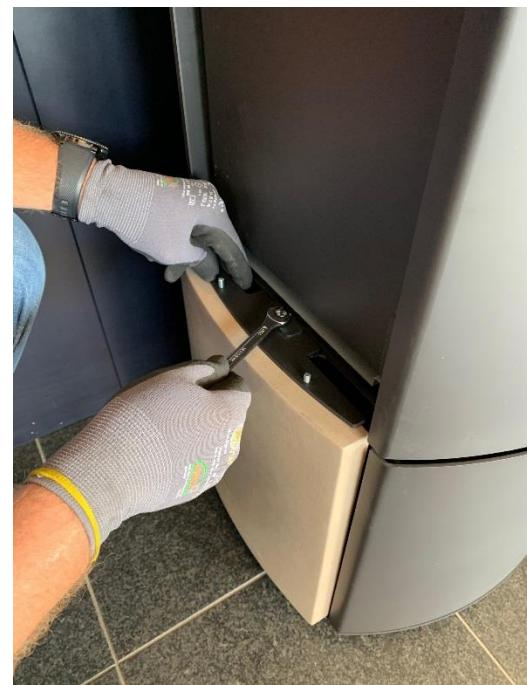
8. Insert the setscrew ends of the second holder into the ceramic and first hand-tighten the holder to the stove.
