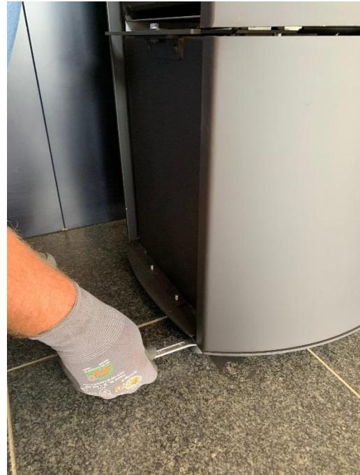
3. Use the height adjusters in the base of the oven for alignment. These can be adjusted with a spanner, size 13.
