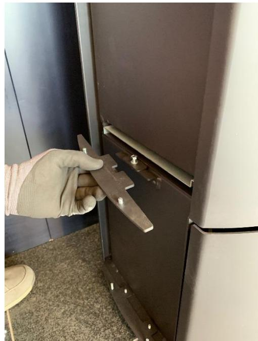
6. Now loosen the screw connection of the second holder and put it aside. Loosen the two fixing screws of the lower holder (underneath the stove) only slightly.
