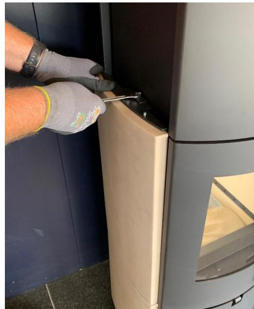
11. Repeat steps 7 to 9 when attaching the middle ceramic element. Carefully check that the door can be opened completely - if not, the position of the ceramic must be corrected accordingly.
