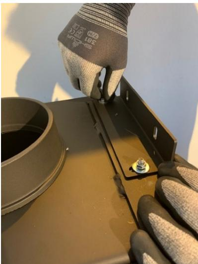
15. Fix the two supplied mounting brackets at the top of the stove on the right and left - hand-tight at first.
