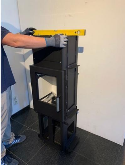
1. Place the stove in its future location before installing the ceramic attachments.
