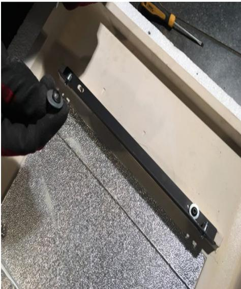
20. Now fix the holding rail supplied with the stove to the back of the front tile. Use the screws (M6 x 16) and one washer each.
