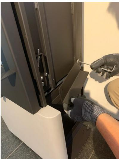
6. To install the first lowest side tile, remove the fixing screws of the pre-assembled steel angle.
