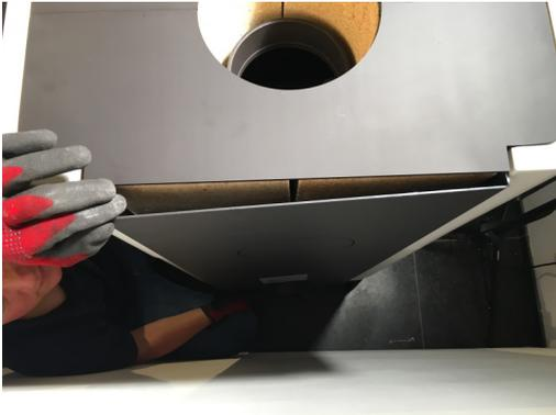
27. Finally hang up the rear panel and fix it with the screws (M5 x 10).
