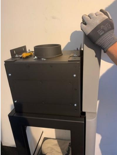
16. Now place the third side tile (with the rounded side to the back) on the threaded rod ends of the angle below.
