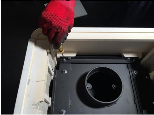
22. By screwing the setscrews in and out of the holding rail, the front panel can be aligned in height so that it is flush with the side panels.
