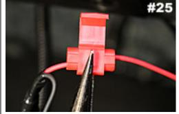
Slide wires in place and use pliers to squeeze metal tap down.
