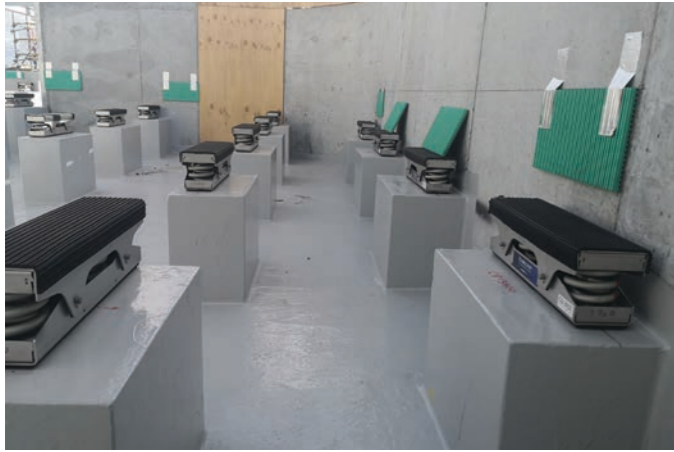
Figure 4. Pre-compressed spring mounts
