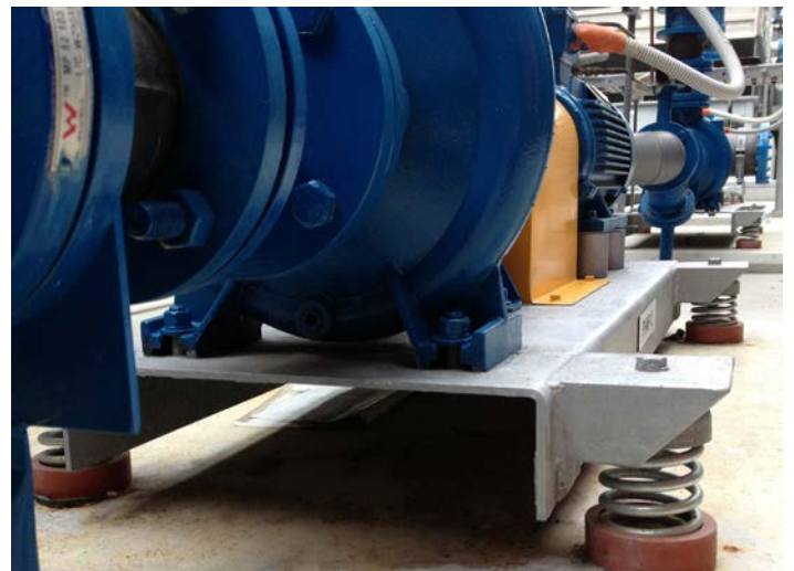
EXAMPLE OF OPEN SPRING ISOLATION
