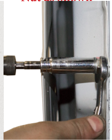
Tighten Rivet Nut as Shown
