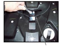
Step 7: Turn Seat Upside Down. Place Bottom T-Bar in place. Holding on Tube on Inside Bar. Push on Inside Bar to Line up Holes through T-Bar, Seat Base and Inside Bar. Insert Bolts Furnished Bolts, through Lock Washer, Bottom T-Bar, Seat Base and into Inside Bar threaded holes and tighten. Helps to use Phillips screw driver that fits in threaded holes, in Inside Bar, to line up one hole, while you insert bolt in the other hole.
