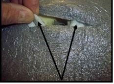
Step 6: Move white pad with wire in it, away from hole both sides.
