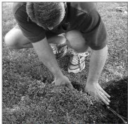
Wires are pushed firmly into the trench.
