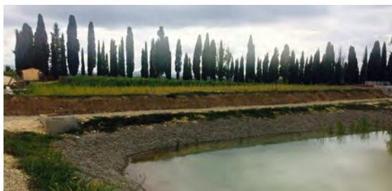
New wastewater treatment plant setting
