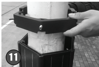
11 Put second brackets over the module in opposite direction to the bottom brackets. Install it in the same way as installing the first brackets.
