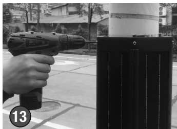
13 Fasten the 6 pieces screws with driver carefully.
