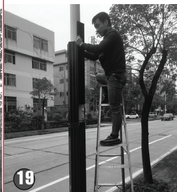
19 Put the second sub module on the bracket in the same way as mentioned in 7. Repeat steps 8, 9, and 10 to complete the pending installation. Finally connect the last two MC4 connectors on top of pole to solar light head directly.
