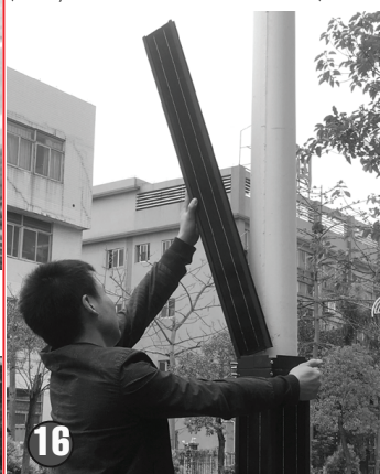
16 Put the second master module on the bracket in the same way as 6 mentioned.
