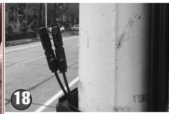
18 Connect the MC4 connectors and put it back inside of the module tube. (It will be invisible from outside.)
