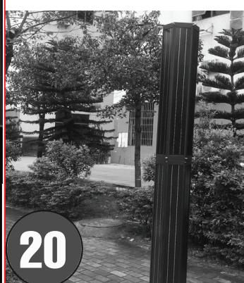
20 SOLAR CYLINDER INSTALLATION COMPLETE
