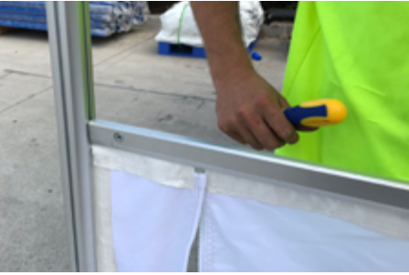
7. Insert the Wall Strip Keder into the Half Wall Bar. Insert the Half Wall Support Bar into the Tracking of the Upper Leg of the Canopy.
