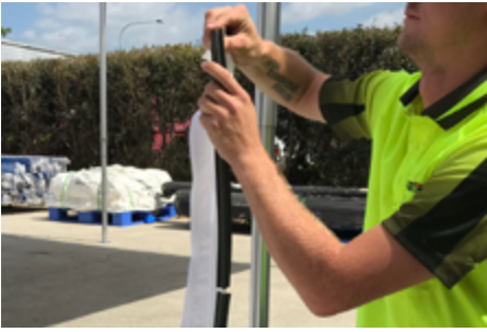
2. Slide the Leg Rubber Inserts (2) along the Keder of the of the Wall Strips. Align to the bottom of Wall Strip.
