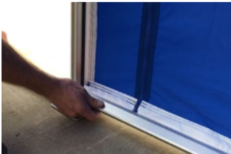
9. Bottom of Full Wall. Insert the Full Wall Keder into the Support Bar and slide Bar along fabric.
