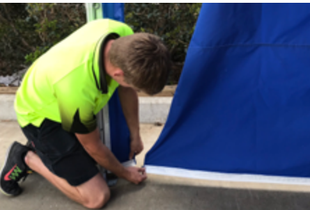
7. Zip the Wall Strip and the Wall Panel together. Repeat on other side.
