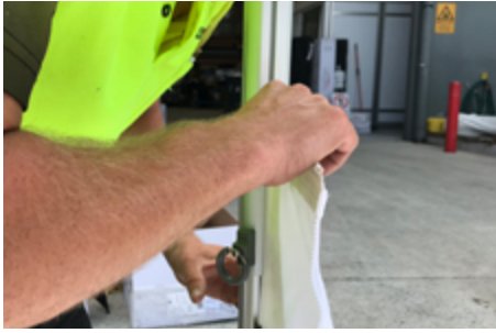
3. Insert the top section of the of the Wall Strip Keder into the tracking of the Upper Leg of tent.
