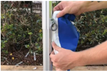
3. Insert the top of the Wall Strip Keder into the tracking of the Upper Leg of Canopy. (Hook facing inwards)
