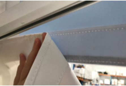
4. Attach the top of the Wall Strip to the roof along the Velco strip. Repeat on other side.
