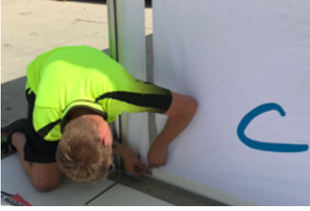
11. Zip the Wall Strip and the Half Wall Panel together.
