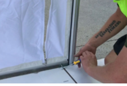
10. Adjust the Half Wall Bar as need to be level and in desired position, tighten bolts to secure.
