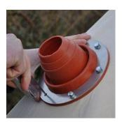
Next, go outside the tent and attach the flashing kit by hanging the first ring and silicone collar on the outside of the canvas (see picture) Push through the bolts from the outside. Go back inside the tent and clamp the second ring on the inside using the nuts provided.
