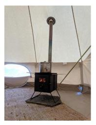
Push the double insulated section through the flashing from the inside. It may help to use a little water and dish soap to lubricate the flue and make it easier to push through.
