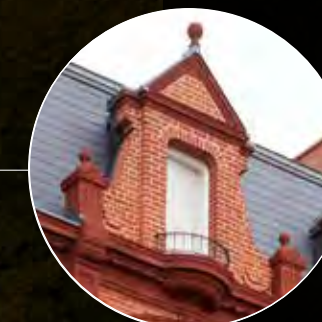
NOTABLE MANSARD ROOF
