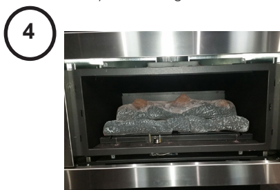
Fit the number 3 log next on the rhs of the middle row.
