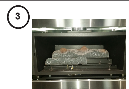
Fit the number 2 log next on the left hand side middle row
