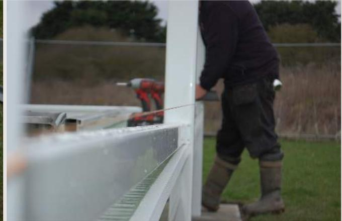
Now string a line between the 2 outside posts level with the top of the brackets, this will make sure the handrails are level all the way through
