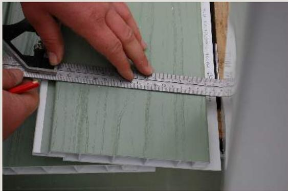
Use a square and pencil to mark your boards and cut with a jigsaw for ease, insert a screw at each joist.
