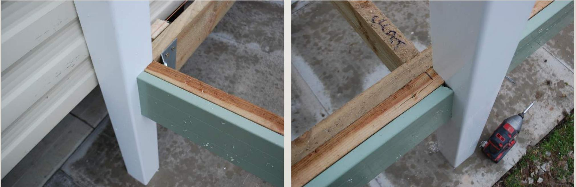
Cut using a fine tooth hacksaw. Cut one end at an angle to achieve a perfect fit and screw from behind
