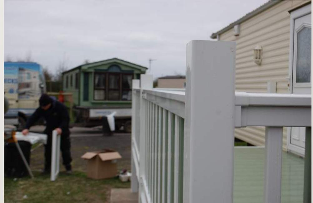
Your rails can then be centered and fixed in place with 32mm stainless steel screws
