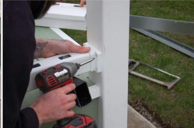
Set the height of the bottom rail up to 100mm max from the deck to the bottom of the rail. Only attach the brackets to the 2 outermost posts using 32mm stainless steel screws
