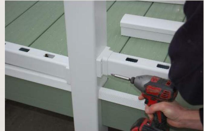
Attach your bottom rail brackets to the centre post using 32mm stainless steel screws
