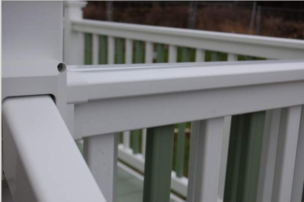
Line up with other top rails, attach top bracket first and the bottom will naturally find its place and can be attached with 32mm stainless steel screws
