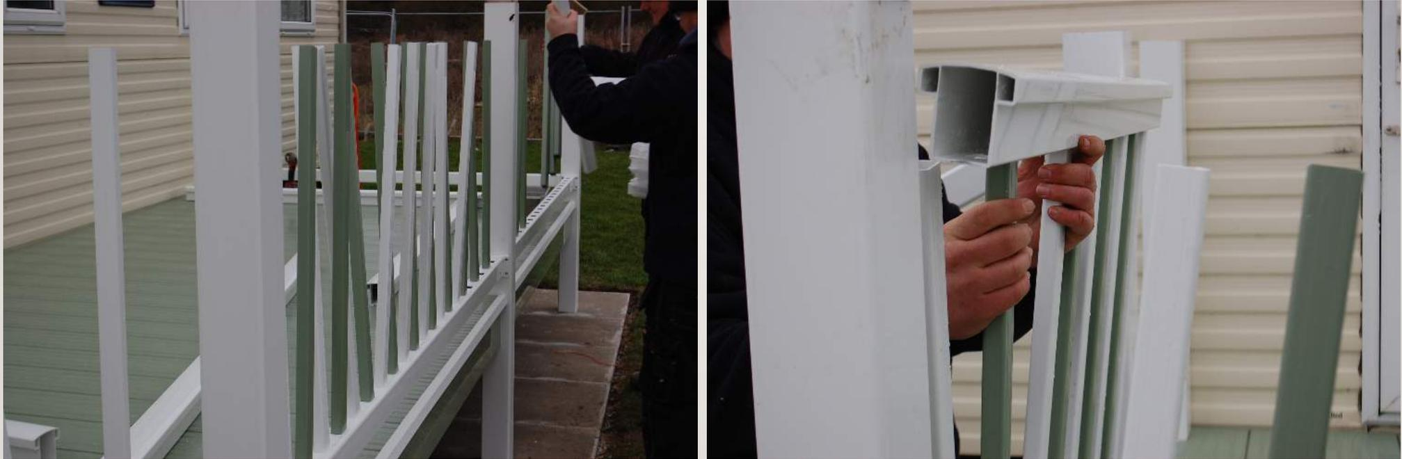
Angle the top rail slightly when inserting the pickets will make this stage easier
