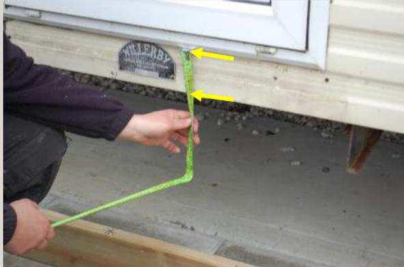
Measure from bottom of door to bottom of home, halve this measurement and deduct the thickness of your chosen deck board and make a note of this.
