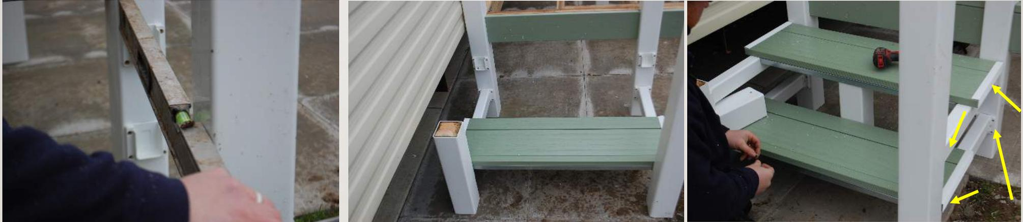
Transfer bracket height across to outer posts using a spirit level, this will keep the the step treads level if the floor is not. Attach brackets and fit step treads as per images above. Cut to size and attach with screws a centre support post to each galvanized step tray. Pilot and screw through the side of each "U" bracket as marked by the yellow arrow on both sides of the step .
