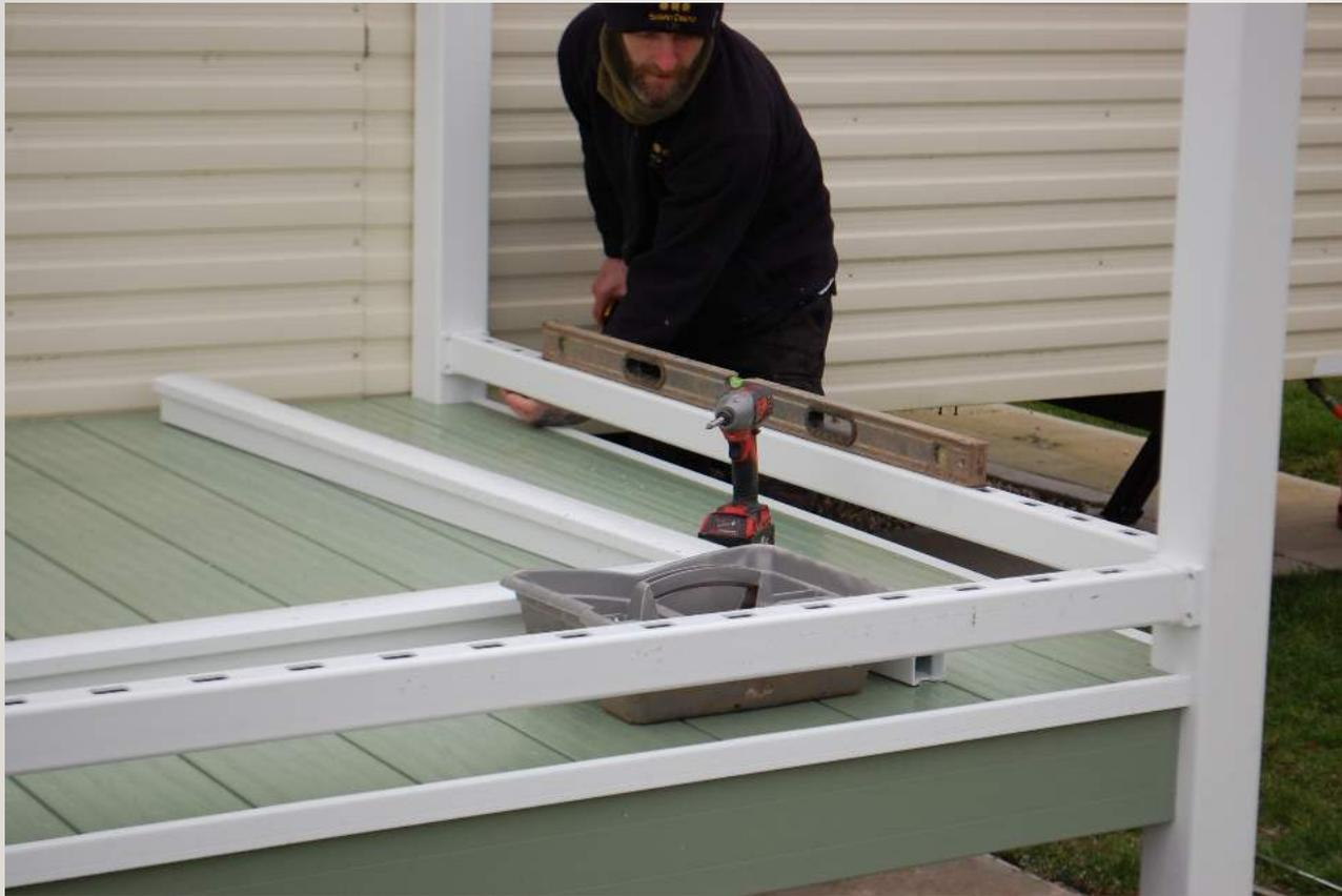
Level up the return rails using a spirit level. Bear in mind because of the fall on the deck the gap will not be exactly parallel.
