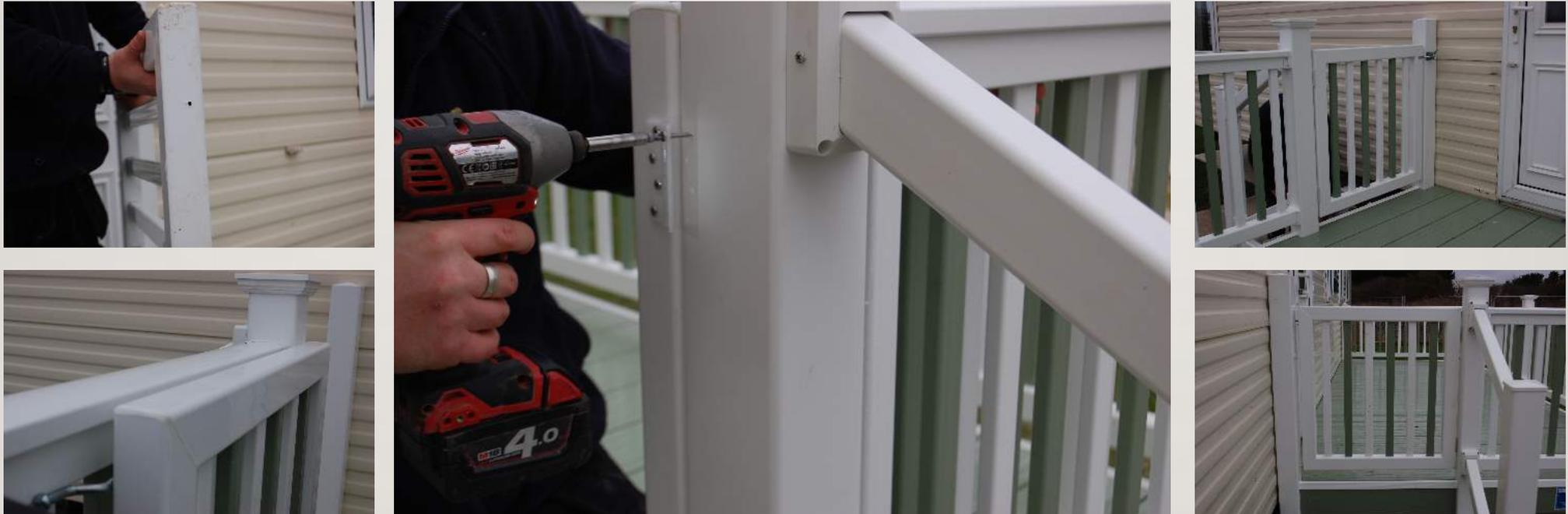
Firstly turn the gate upside down and drill 3 5mm drain holes. Next line the gate up with the top rail and then screw the hinges in place. Finally attach your latch and check operation.
