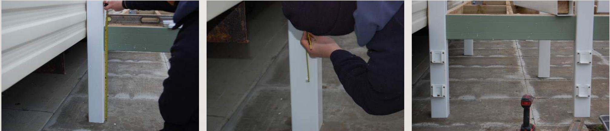
Measure from the top of the frame to the floor and divide this measurement by 3 and mark the post. i.e. if the measurement is 600 each mark will be at 200mm distance. Use a square to mark the post across, place the top of the bracket to the mark and attach to the post with screws.
