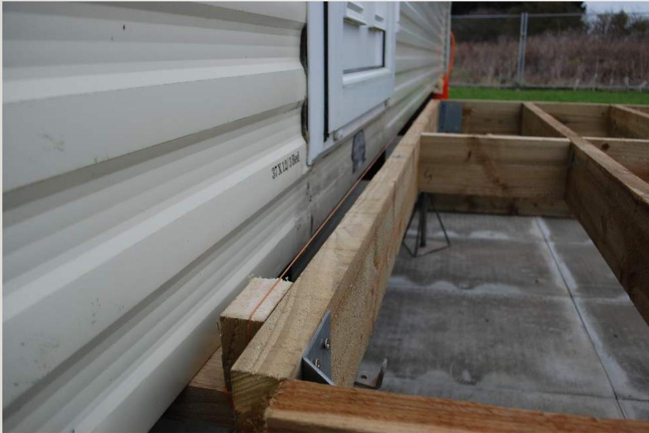
The frame/s can now be set to the string line, we use caravan axle stands to hold the frame/s to the correct level as they are easy to adjust.
