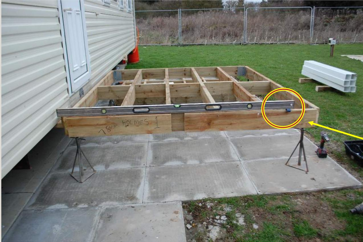
Allow 15mm fall using an 1800mm spirit level away from your van, we use 3 x 5mm packers. This is to allow for water run off.
