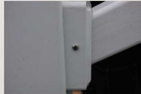
Attach bottom rail brackets and rail with 32mm stainless steel screws.
