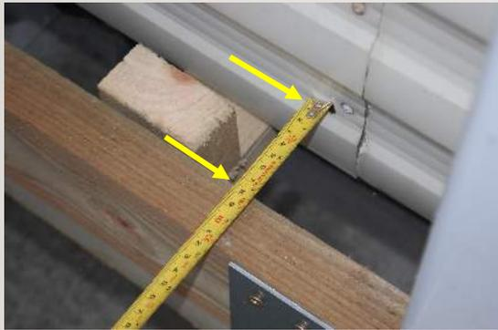
These “L” shaped brackets need to be set approximately 70mm from the front of the home to the face of the timber and can now be screwed to the bottom edge of the home.
