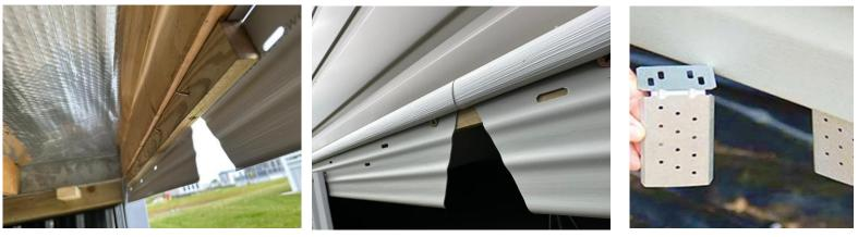
A wooden batten can be used, slightly off set from the edge underneath so the Top Trim Back is flush with the side of the home. **Do not screw directly to side of home**. Alternatively, we offer galvanised skirting brackets on our website.
